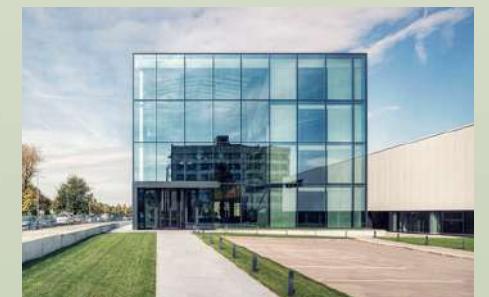
Figure 6 : Window glaze exterior
